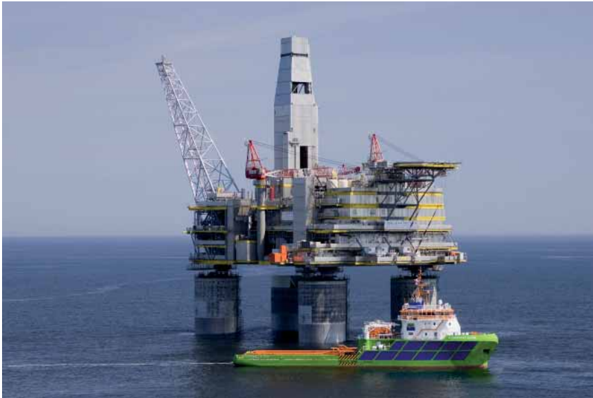
Figure 2: Lunskoye-A Production Platform, installed summer 2006 (Source: Sakhalin Energy Investment Company)
