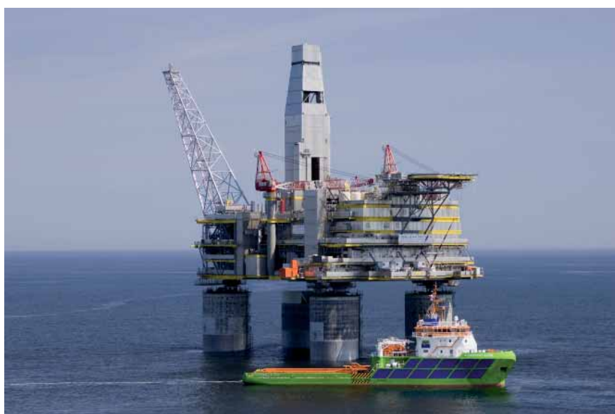
Figure 2: Lunskeye-A Production Platform, installed summer 2006 (Source: Sakhalin Energy Investment Company)
