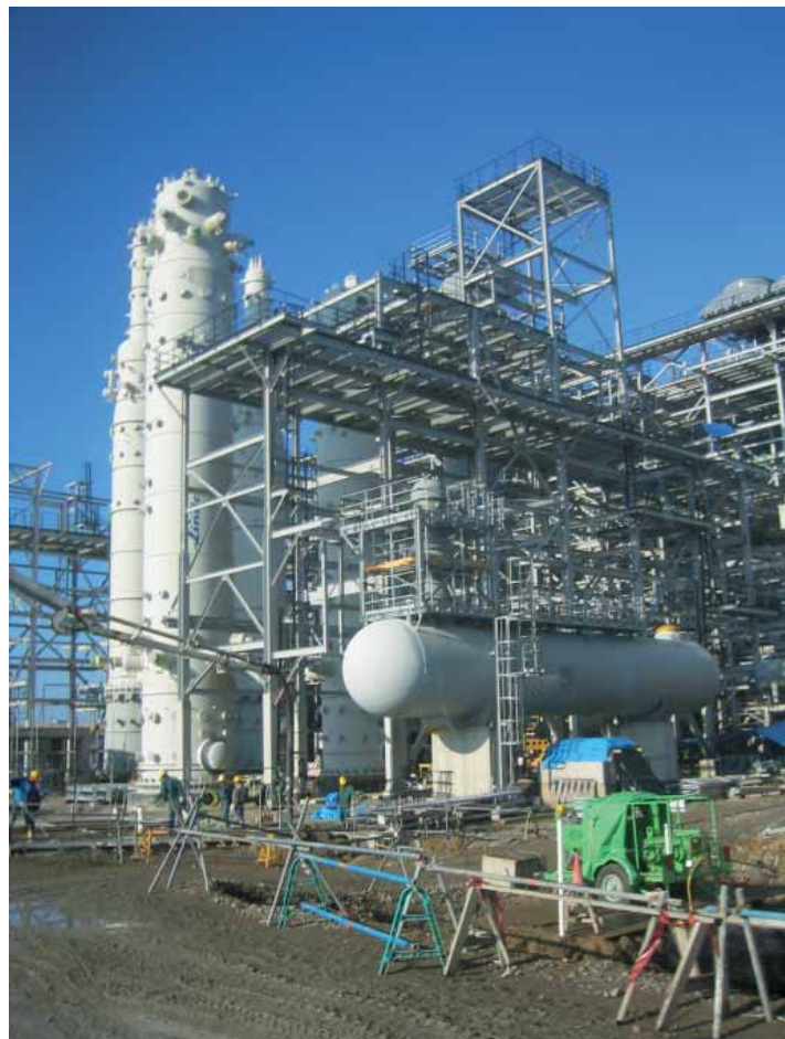
Figure 1: Construction work at the LNG Site (Source: Author).
