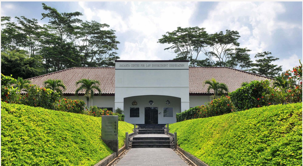
Photo of the JCLEC building in Semarang, Indonesia. Photo courtesy of the JCLEC.
