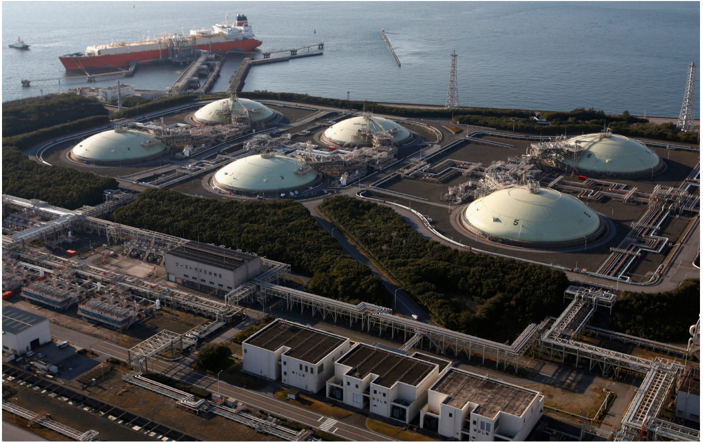
Liquefied natural gas (LNG) storage tanks and a membrane-type tanker are seen at Tokyo Electric Power Co.'s Futtsu Thermal Power Station in Futtsu, east of Tokyo, February 20, 2013. Japan's imports of LNG hit a monthly record of 8.23 million tons in January, on an increased need for fuel to generate electricity after the nuclear sector was hit by the Fukushima crisis, customs-cleared Ministry of Finance data showed. REUTERS/Issei Kato
