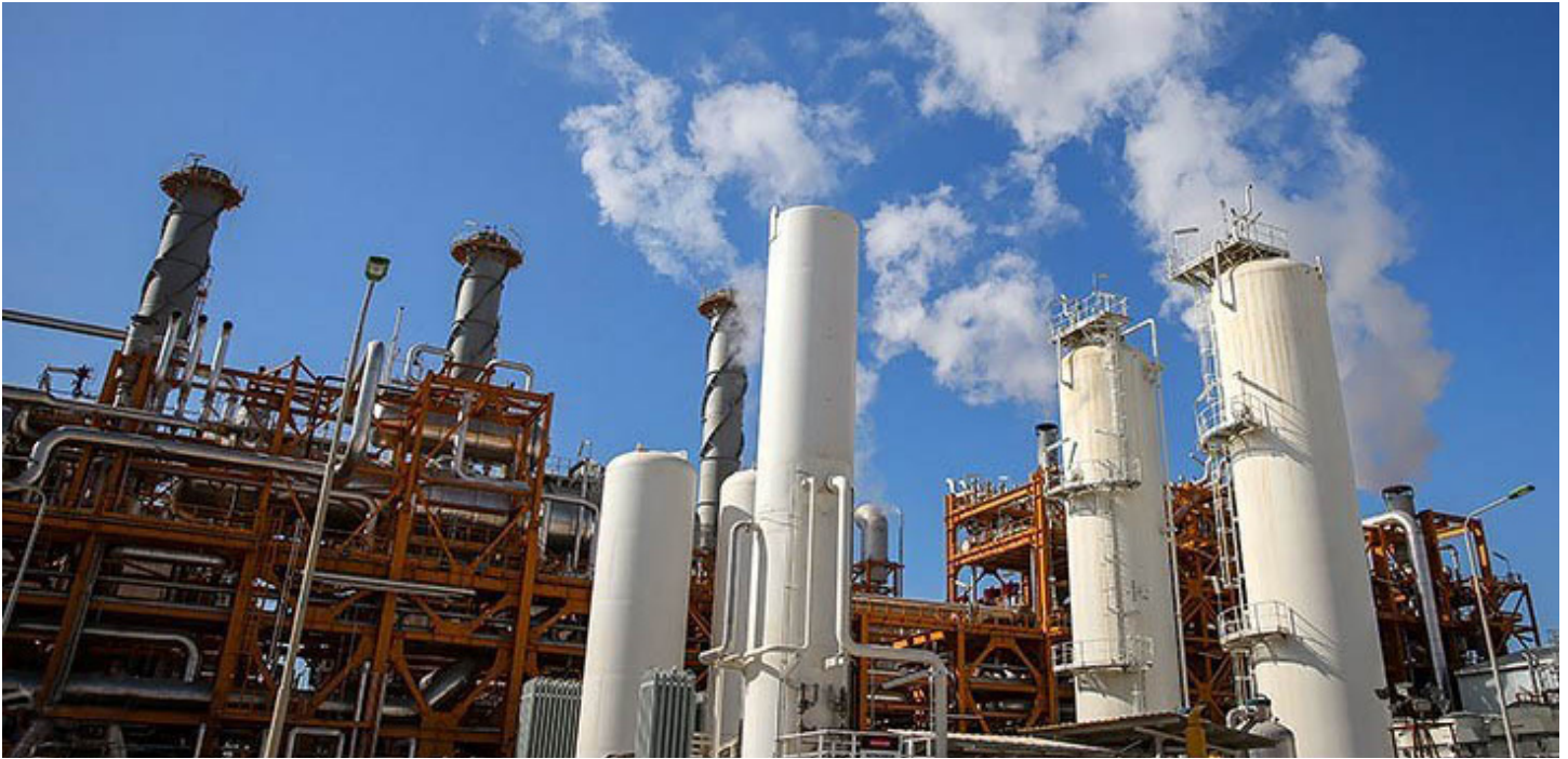
South Pars Onshore Facilities near Asaluyeh City, December 11, 2013. Photo: Wikimedia Commons, Hamed Malekpour
