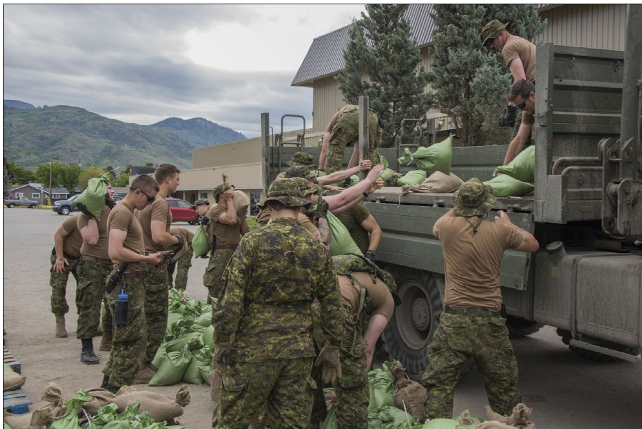
Canadian Armed Forces members from CFB Edmonton assist in dyke building and sand bagging during Operation LENTUS 18-03 in support of flood relief efforts in Grand Falls, British Columbia, 19 May 2018.
