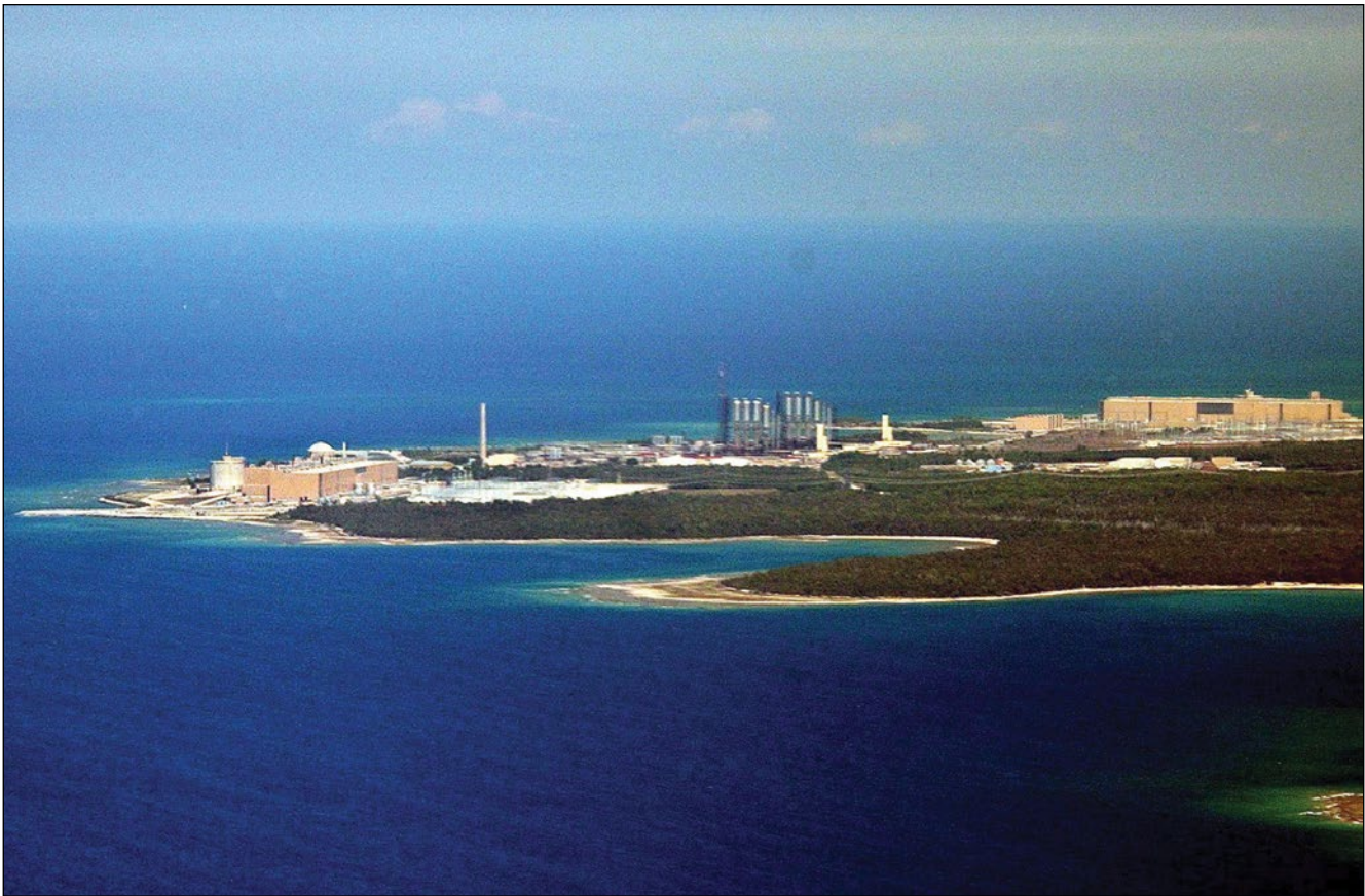
An aerial view of the Bruce Power nuclear generating station in Kincardine, Ontario. An EMP event affecting this facility could have catastrophic consequences.
