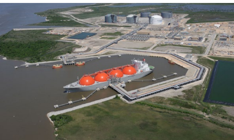
Sabine Pass export terminal in Louisiana is one of four in the United States authorized to export LNG to both FTA and non-FTA countries. In February 2016, the first LNG cargo from the lower 48 states set sail from Sabine Pass to Brazil. (Think Defence/Flickr)
