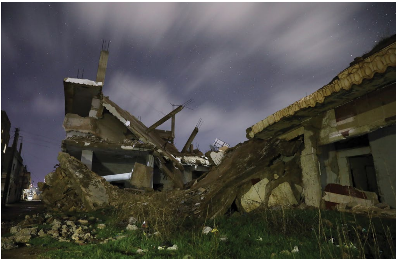
Damaged houses are pictured at night in the city of Dar'a, in southwestern Syria, in February 2018. (Photo by Alaa Al-Faqir/Reuters)
